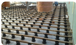
2) Align pedestals with wood battens and Insu@Jac Wood Holder
