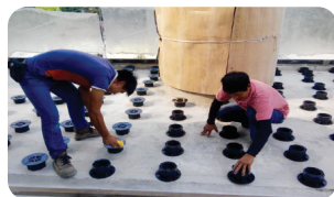
1) Setting out pre-assembled Insu@Jac pedestals
