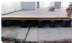
5) Installation of bamboo decking
