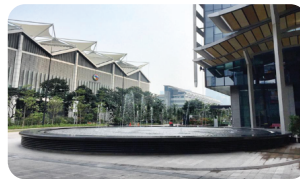
5) Testing the system by filling the fountain with water
