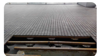
6) Insu@Jac pedestal level raising system below bamboo decking
