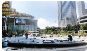
4) Checking completed floor levels
