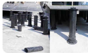
2) Utilising Pipe Extender to achieve raised levels of 95mm to 1500mm
