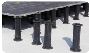
1) Setting out pre-assembled Insu@Jac pedestals
